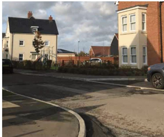
Figure 22: Poor quality public realm with poor surface treatment and maintenance, Biggleswade.
