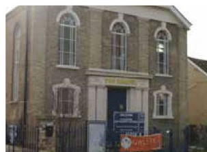
Good level of detail on windows and door frame decoration
