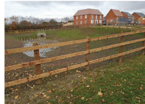
Figure 23: Poorly maintained SUDs in recent development, Langford.
