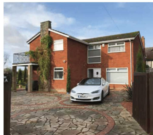
Figure 8: Red brick detached family house situated between the B659 and River Ivel.
