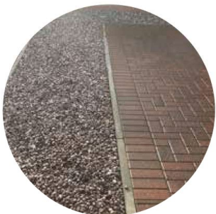
GRAVEL & PERMEABLE CONCRETE BLOCK PAVING
