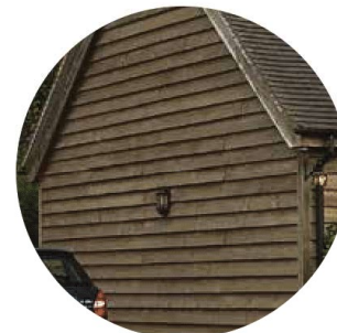
PAINTED TIMBER WEATHERBOARDING
