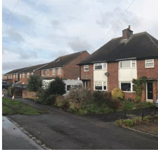
Figure 10: Semi-detached family houses along East Road.
