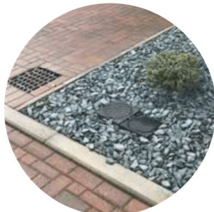
MIXED PERMEABLE SURFACE TREATMENT: CONCRETE BLOCKS & CRUSHED GRAVEL STONE
