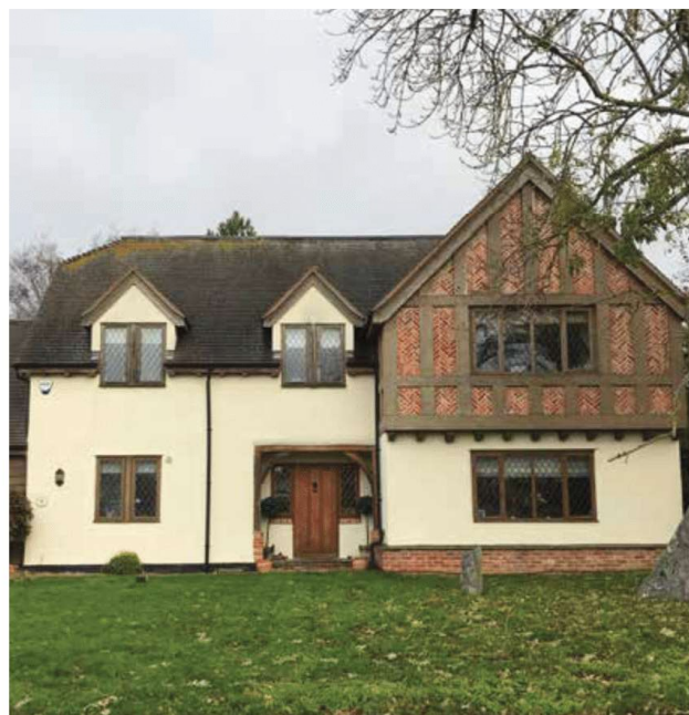
Good level of detail and mix of building material, half timber structure with red herringbone brick detailing.
