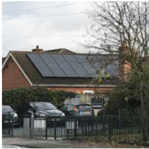
Retrofitted solar panels.
