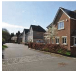
Shared surface/ private drive with quality surfacing, Baldock.
