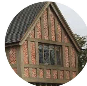
HALF TIMBER FILLED WITH RED BRICKS (HERRINGBONE BOND)
