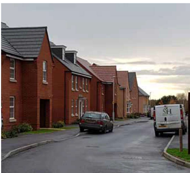
Poor public realm treatment, overuse of red brick, high density, Langford
