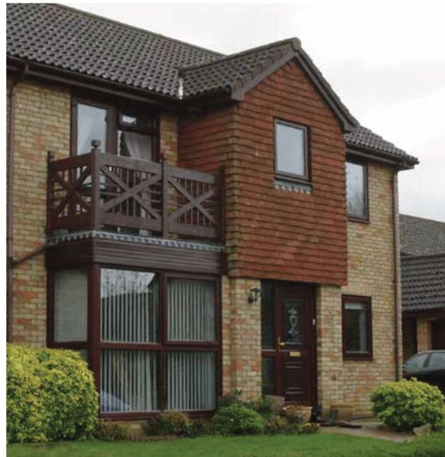
Cul-de-sac development along Old Mill Close, showing a good amount of architectural detailing and mix of building materials.
