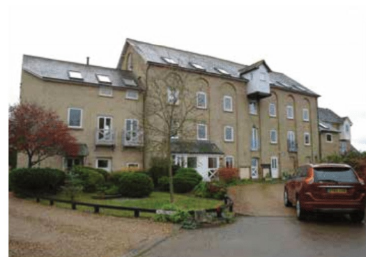
Figure 7: Former corn mill on the River Ivel, converted for residential use.
