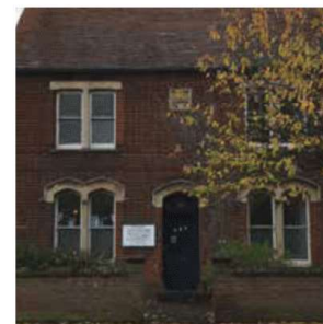
Arch detail on windows and doors.
