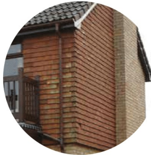
HUNG TILES/ BRICK CHIMNEY
